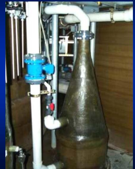
Side flow enters downflow bubble contactor (Marine Biotech) to remove off-gas.
