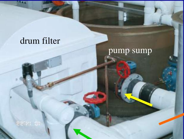
Drain piping should be plumbed to allow drum filter bypass to direct flow to: Drain (away from RAS) • during cleaning events Pump sump • When servicing drum filter drain
